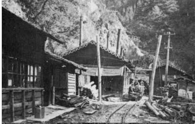
Riding in carriages to enter and exit the vein (Ikuno Silver Mine in Showa Period)
